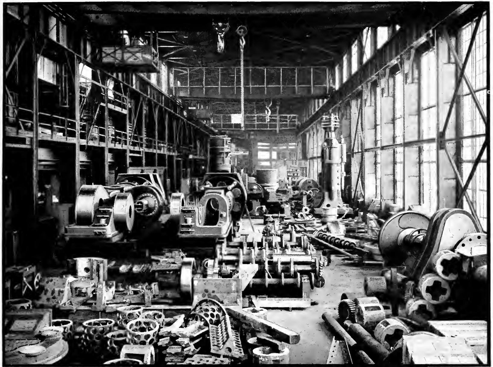
View on Erecting Floor
